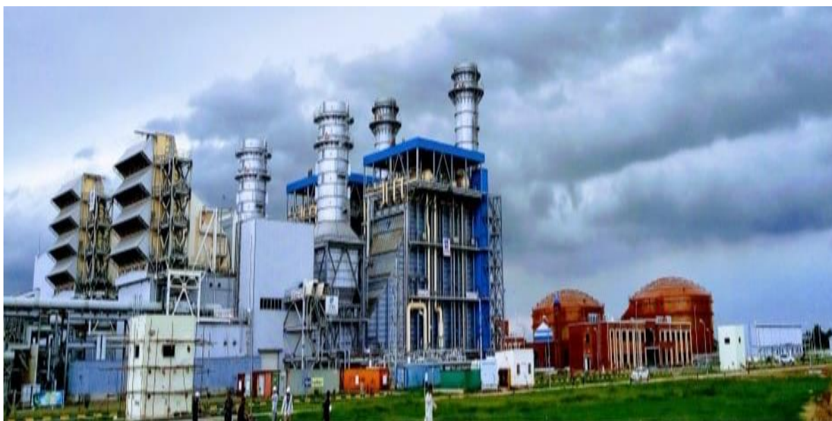
1223 MW Balloki Power Plant
