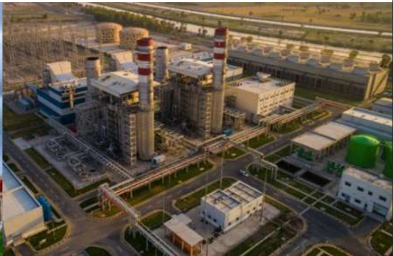
1230 MW Haveli Bahadur Shah
