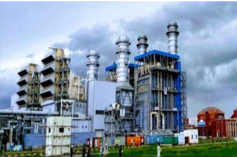
1223 MW Balloki Power Plant
